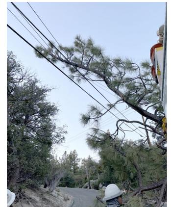
*Inspection photos show tree branches that had fallen onto insulated wires (covered conductors). Power remained safely on for customers in the Idyllwild area of Riverside County-November 25, 2021.
